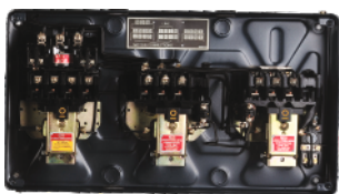
Interior View of MK1 FASD
