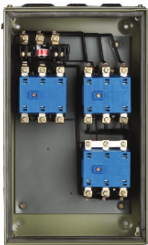
Interior View of ML SASD
