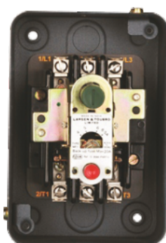
Interior View of MF1 DOL - 3Ø Starter
