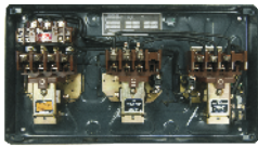
Interior View of MK2 FASD
